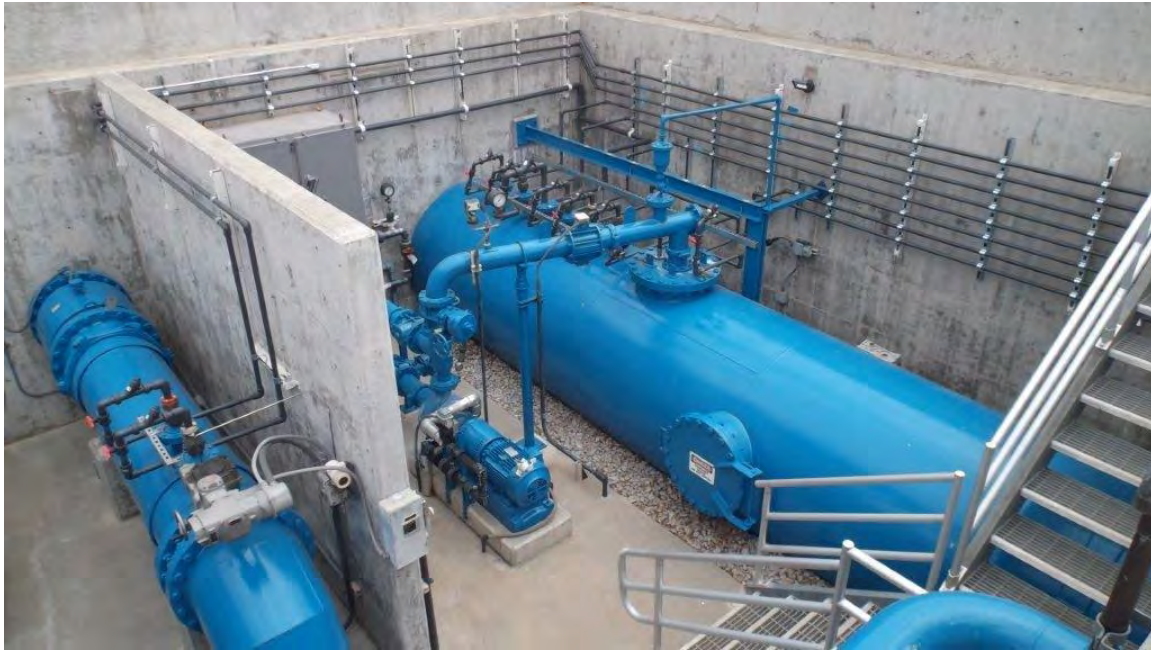
Water Treatment Plant chemical feed piping replacement (May 2017)
