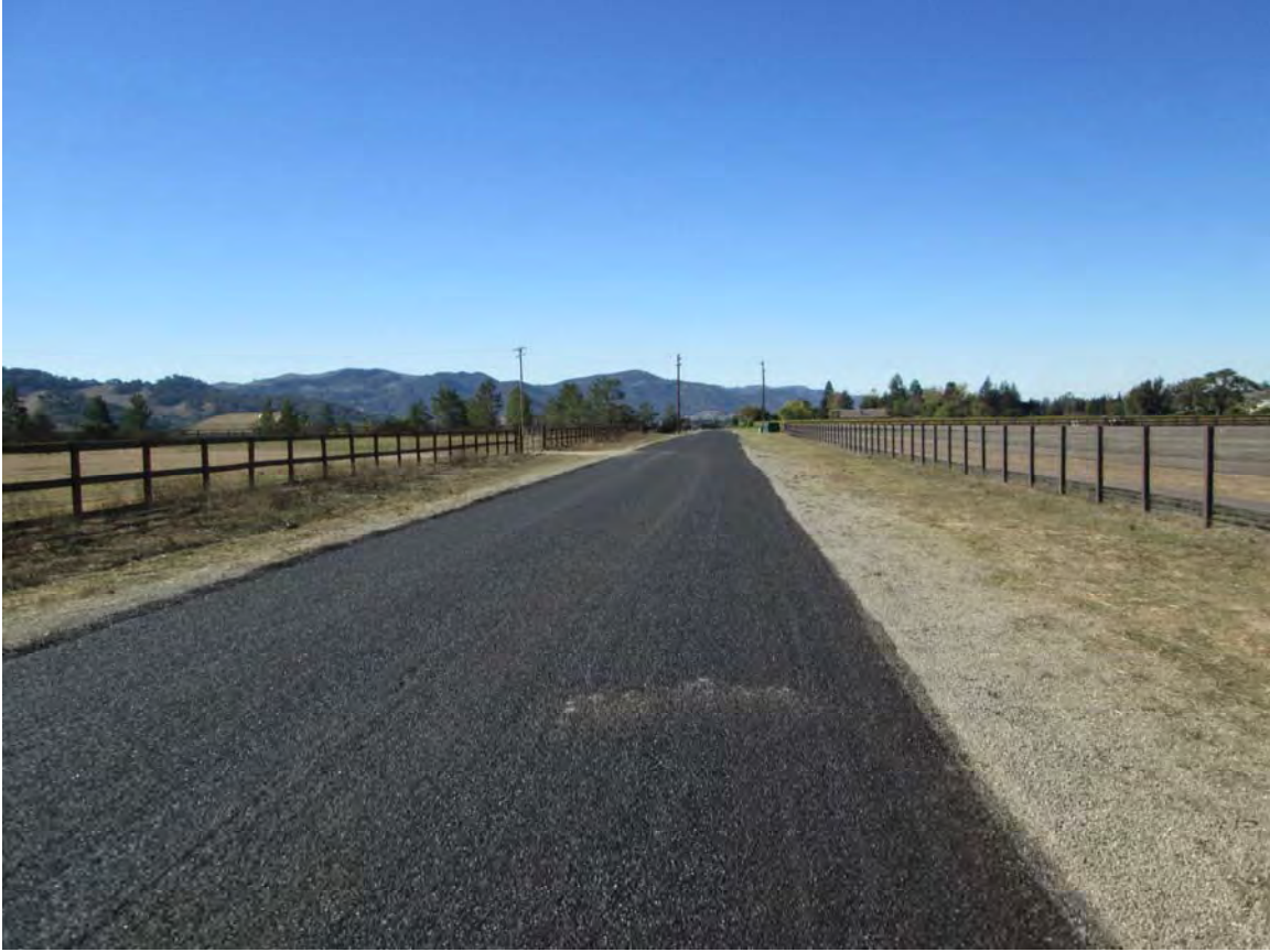
Resurfaced roadway at Santa Ynez Pumping Plant
