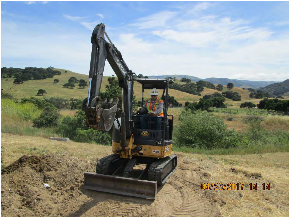
Installation of emergency generator at Tank 7 location
