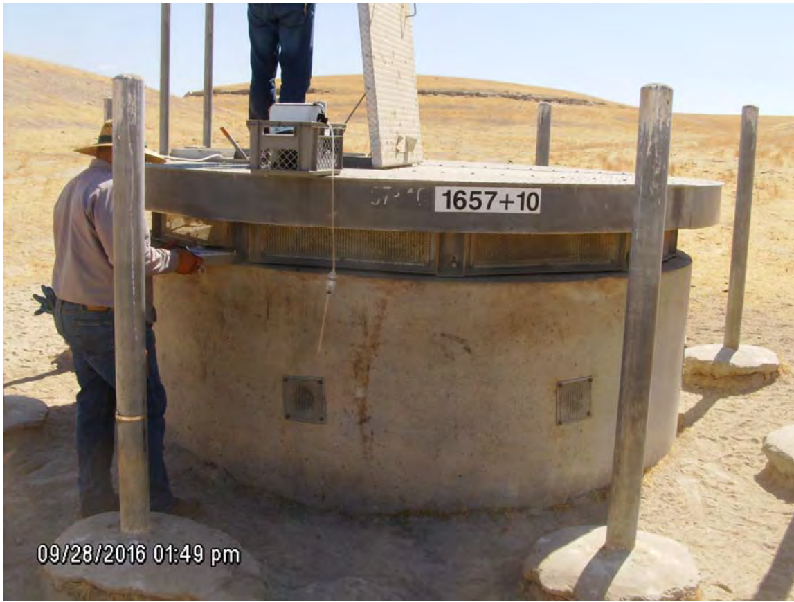
Crew performing vault assessment at AVAR
