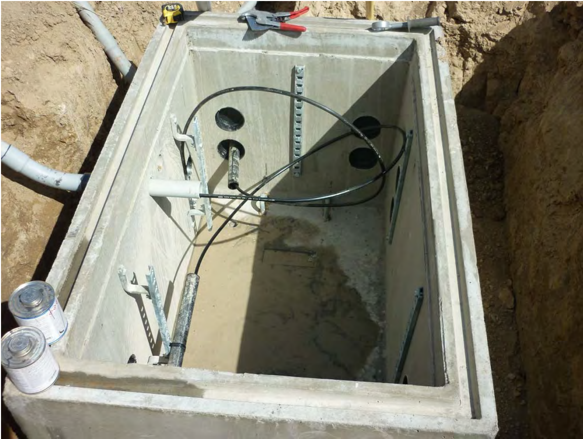
Conduit installation at Shandon Turnout Vault. (April 2017)
