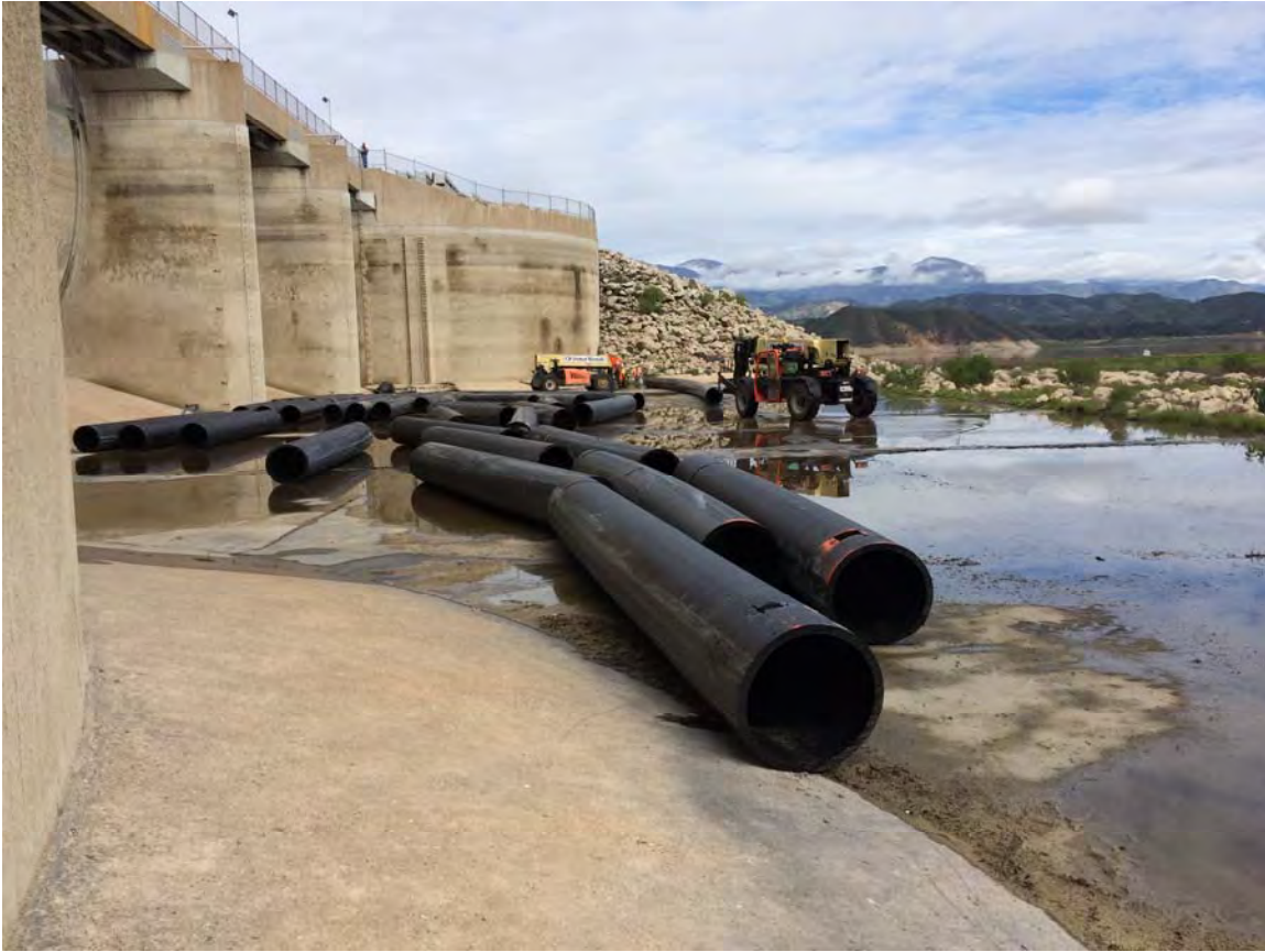
Bypass Pipeline Removal at Bradbury Dam (February 19, 2017)
