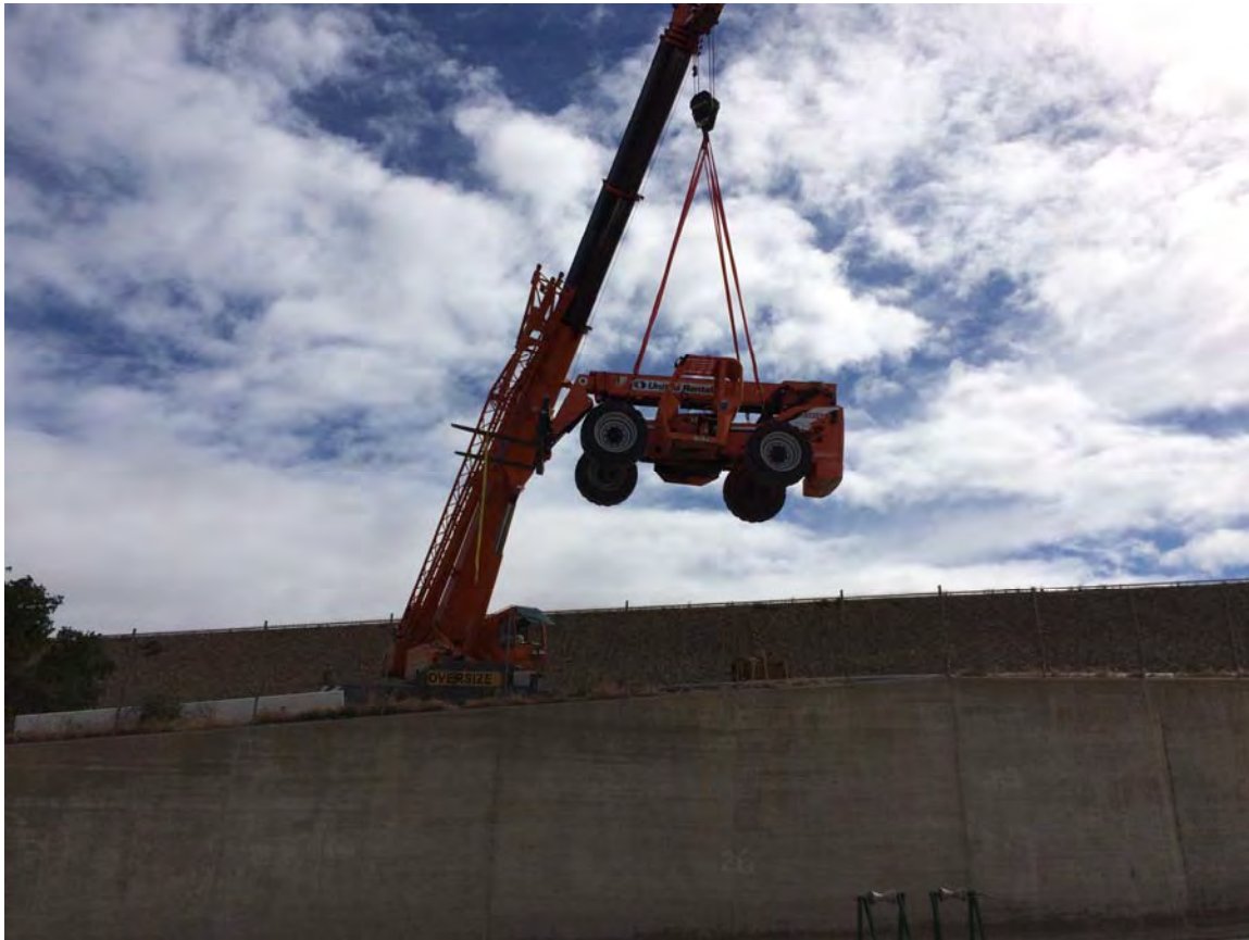
Lowering crane for bypass piping replacement. (April 2017)
